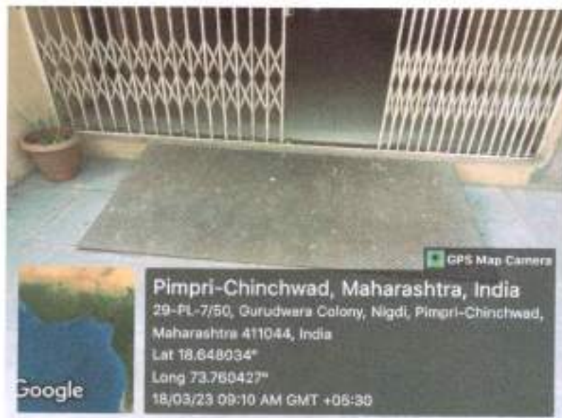
Geotagged photograph of ramp
