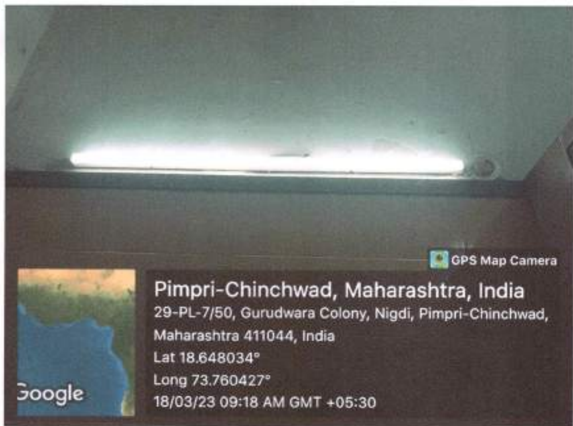
Fitting of dimming Sensor at male toilet Ground Floor
