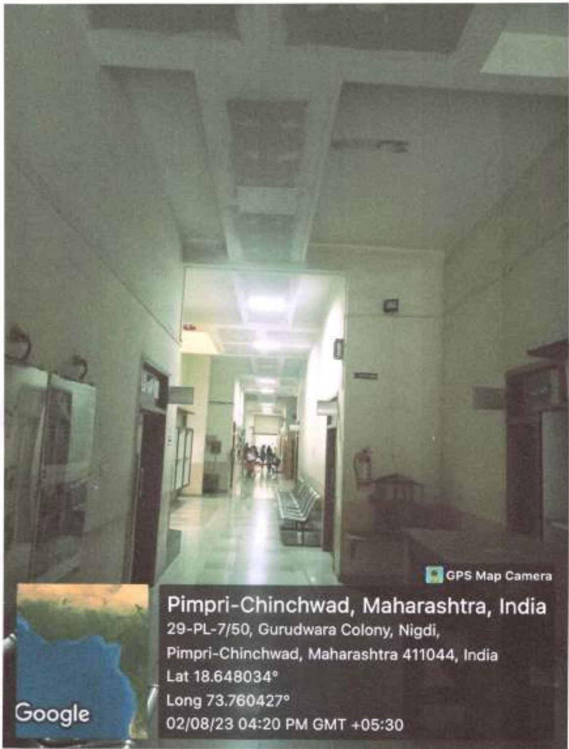
Installation of LED Tube in campus Corridor area.
