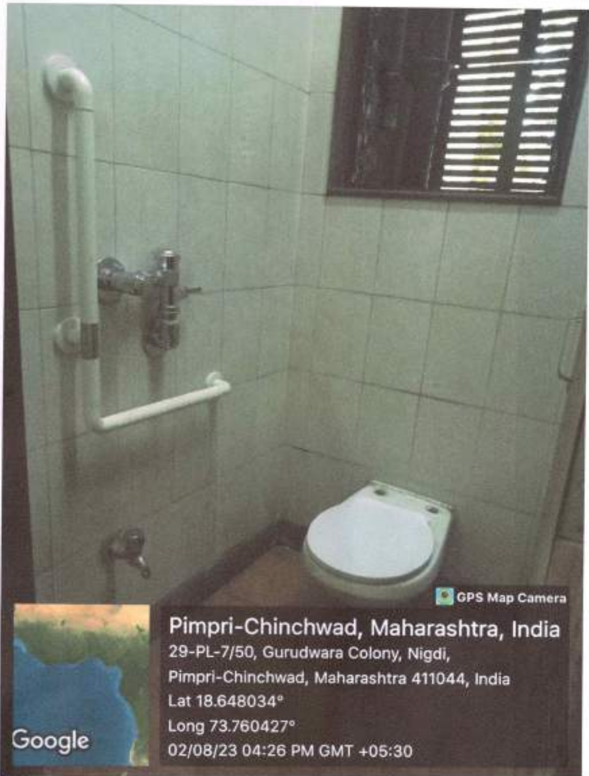
Geotagged Photograph of installation of grab bar at female toilet.
