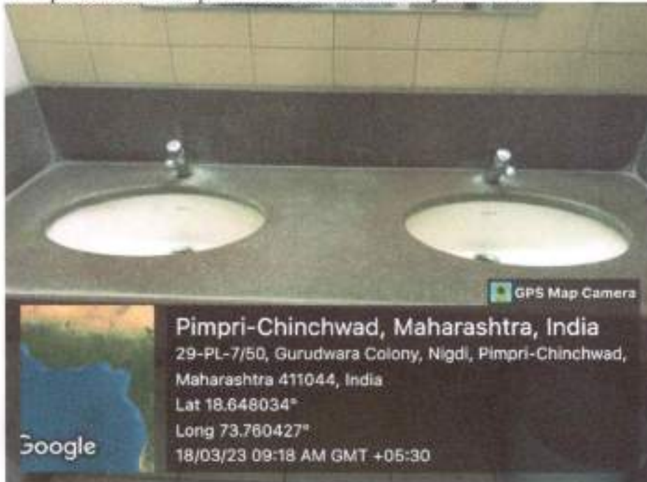
Geotag photograph of Boys Toilet at Ground Floor
