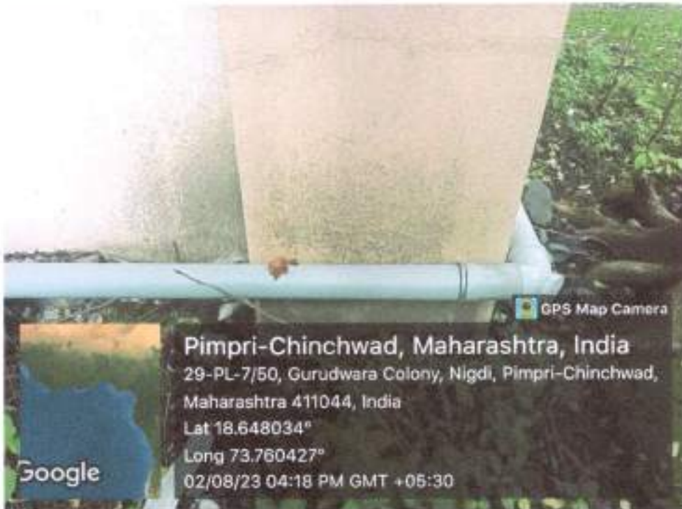
Geotagged photograph of downpipe second location.
