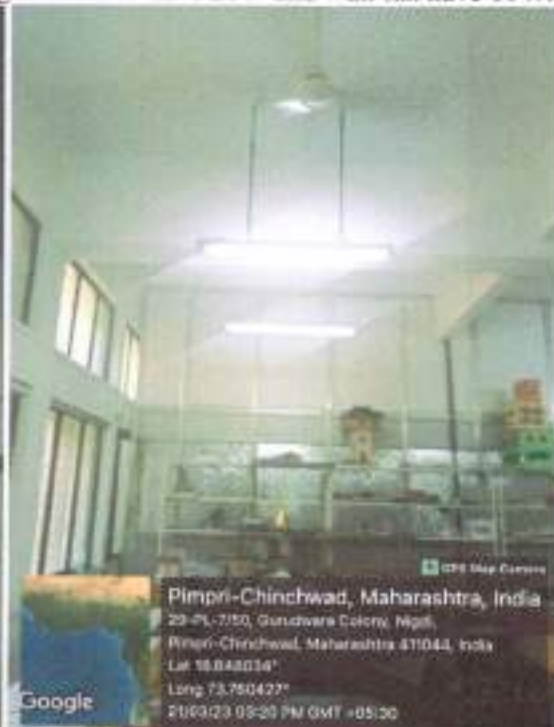
Classroom have replaced LED tube from Fluorescent tube. Power wattage of each tube is 36W.
