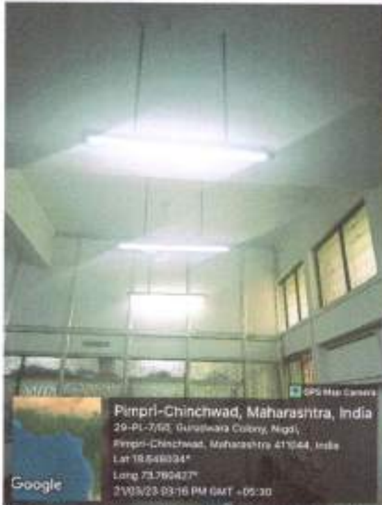
Classroom have replaced LED tube from Fluorescent tube. Power wattage of each tube is 36W.
