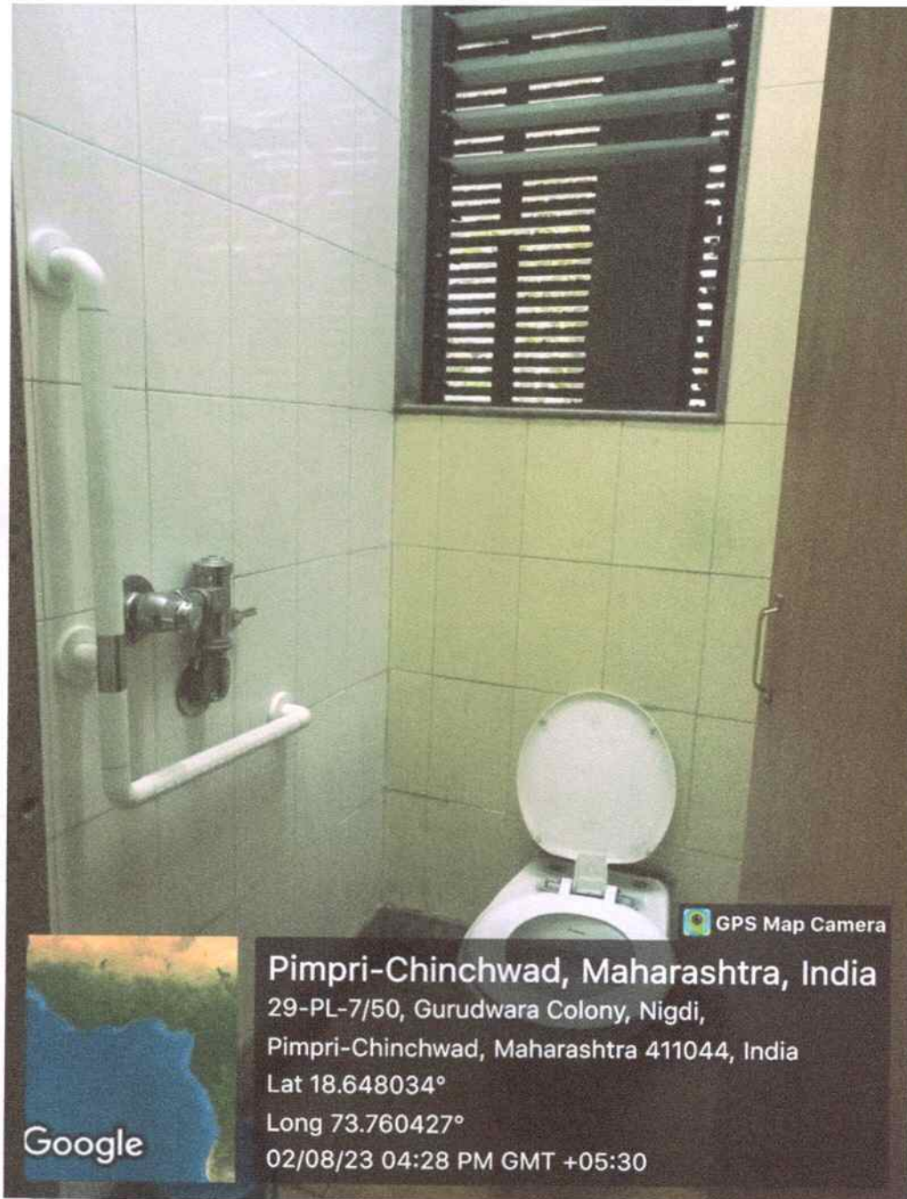
Geotagged Photograph of installation of grab bar at male toilet.
