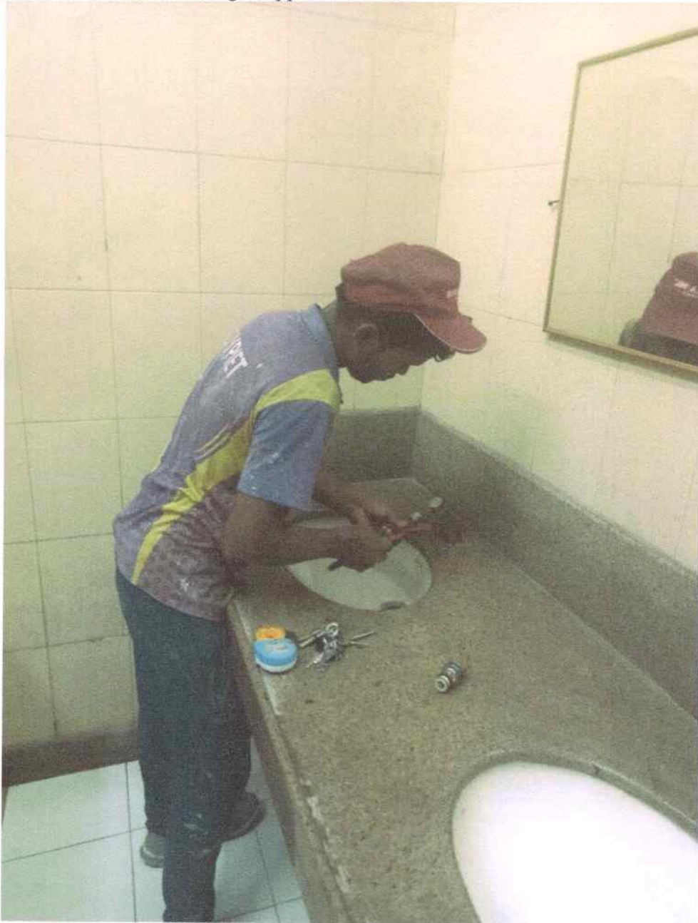
Installation performed by an expert in female toilet at college campus.
