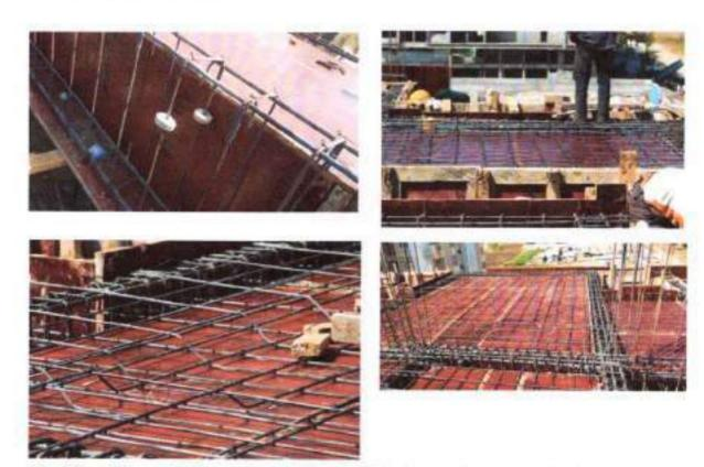
Total load is carried in a direction perpendicular to the supporting beam.
